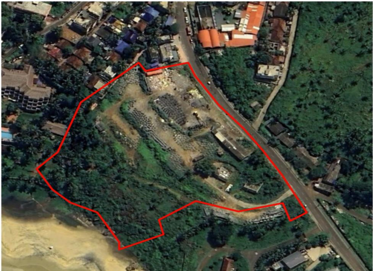
Figure 5 Site Aerial View
